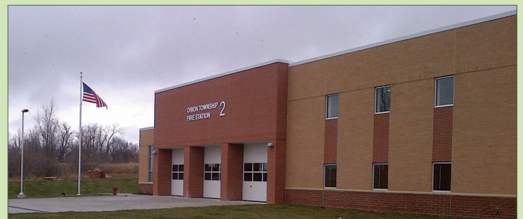
After construction - December 2014
